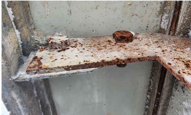
Bolted Steel Plate
