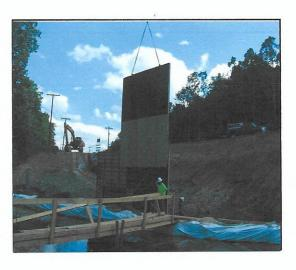
RASTO panels are clamped together to create almost any wall or column dimension. They can also be stepped to accommodate uneven footing or slab elevations.
