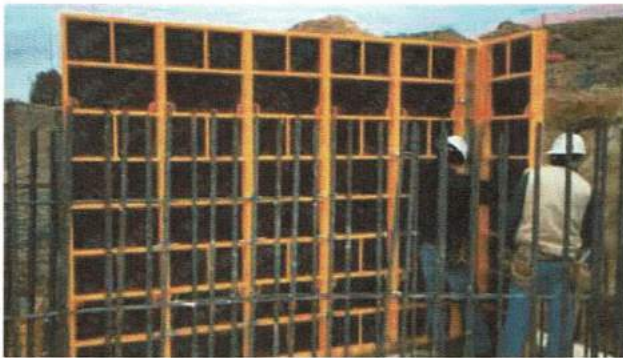
▶ Handset erection of the formwork
