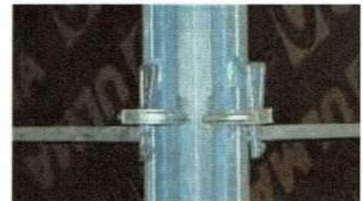
► Fixed clamps on formwork corner
