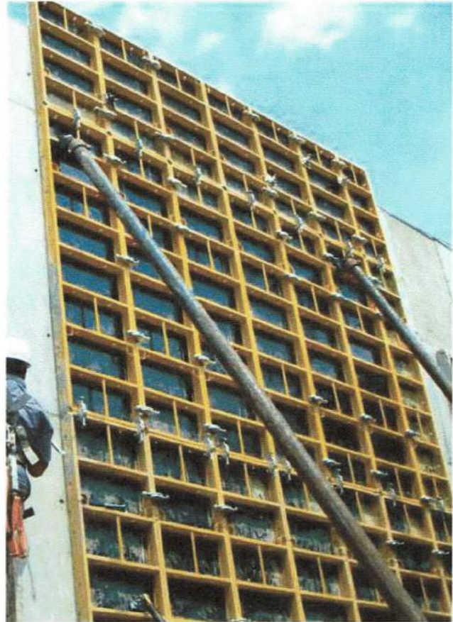
▶ Forming of high walls with formwork gangs
