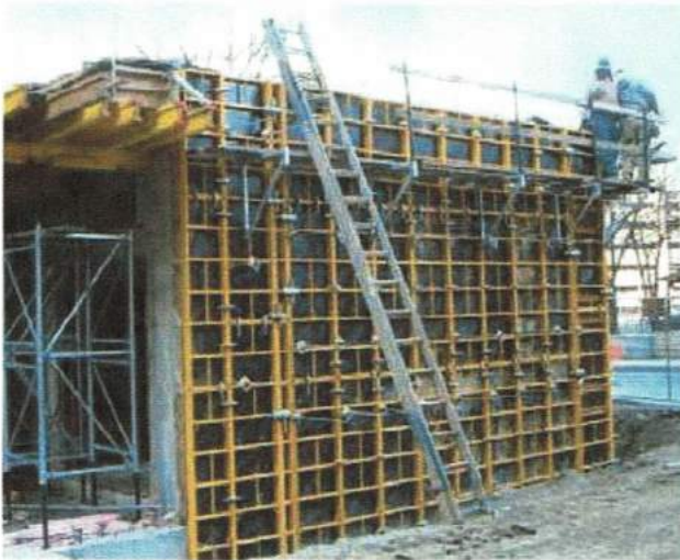
▶ Safe working platforms
