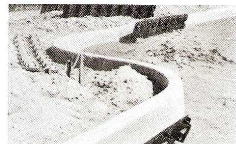
Full height segmented batter face plates are used.
