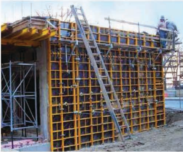
▶ Safe working platforms
