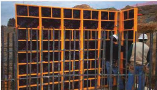
▶ Handset erection of the formwork
