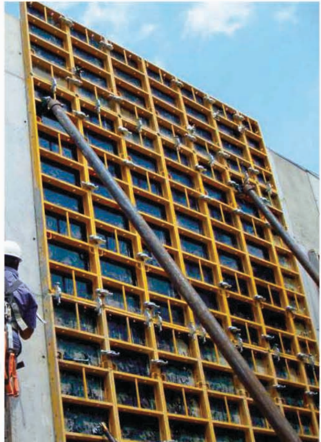
▶ Forming of high walls with formwork gangs
