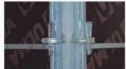
► Fixed clamps on formwork corner
